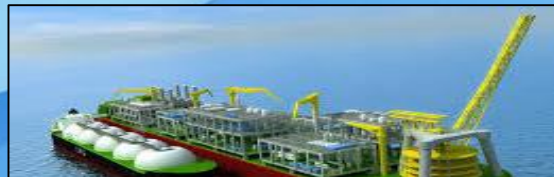
Floating Gas to Chemicals
